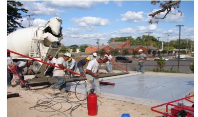
Sponsor: Arkansas Ready Mixed Concrete Association
