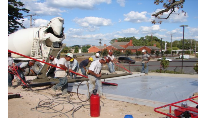
Sponsor: Arkansas Ready Mixed Concrete Association
